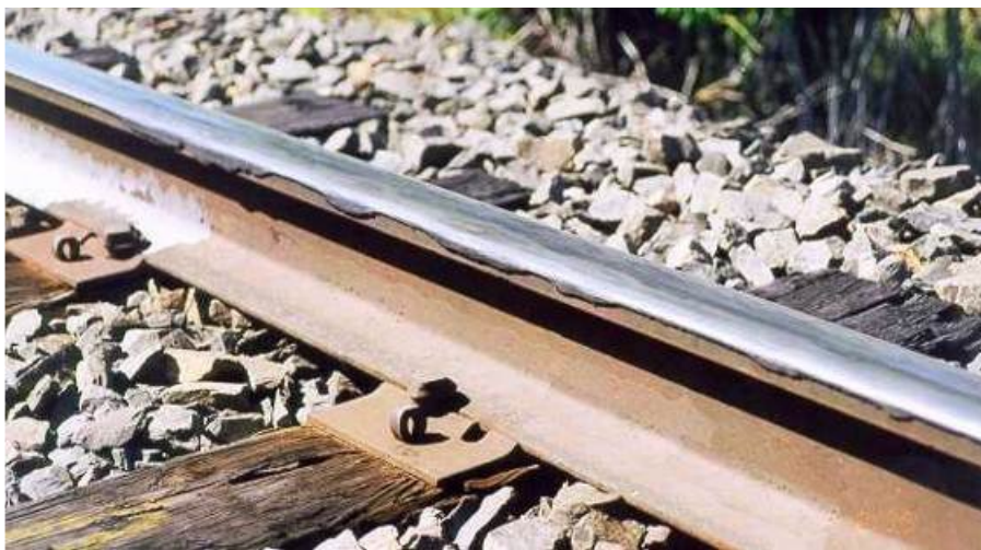
Abbildung 3-4 Rail plastic flow associated with long pitch corrugations (aus [8])
