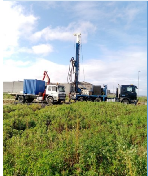
Figure 8. Picture of the Helgúvík injection site in preparation, Summer 2022.
