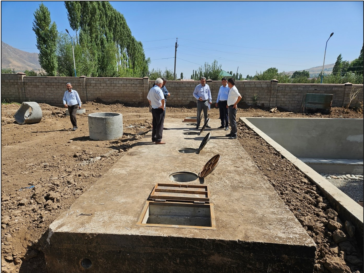
Figure 1: Construction of Decentralised Wastewater Treatment System in Faizobod
