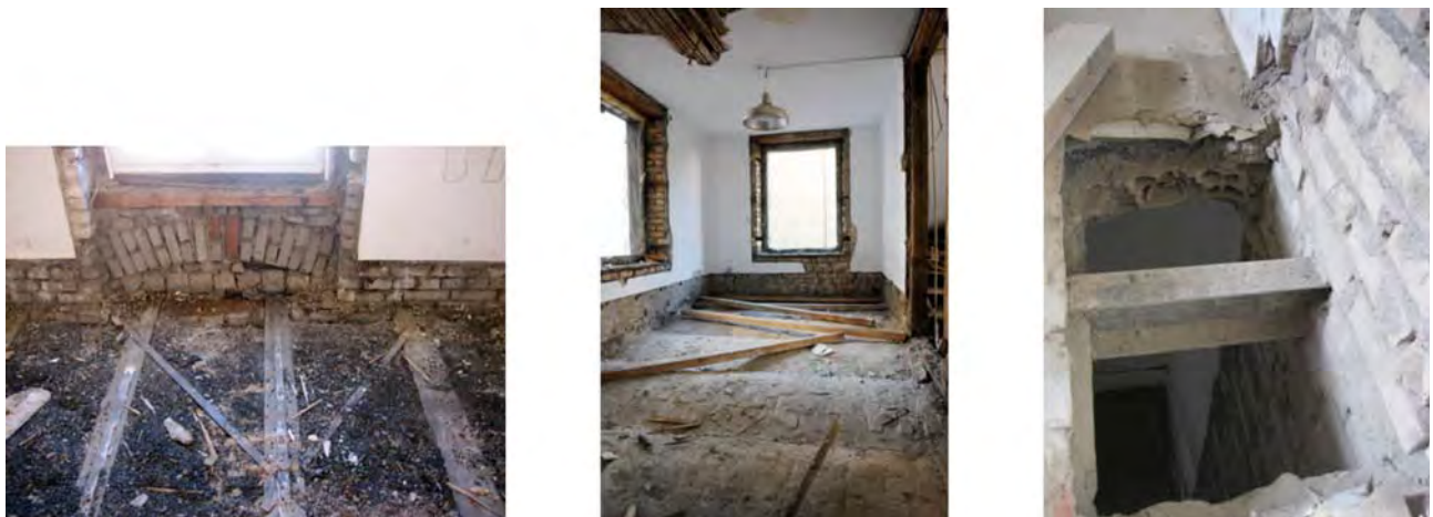
Figure 5: The construction of historical building is often complex and heterogeneous: Wooden beams running to a window alcove with a filled discharging brick arch. Grouted anchors of iron
