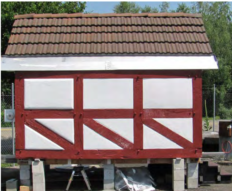
Figure 17: Retrofitted historical timber frame test wall for long term testing under real climatic conditions
