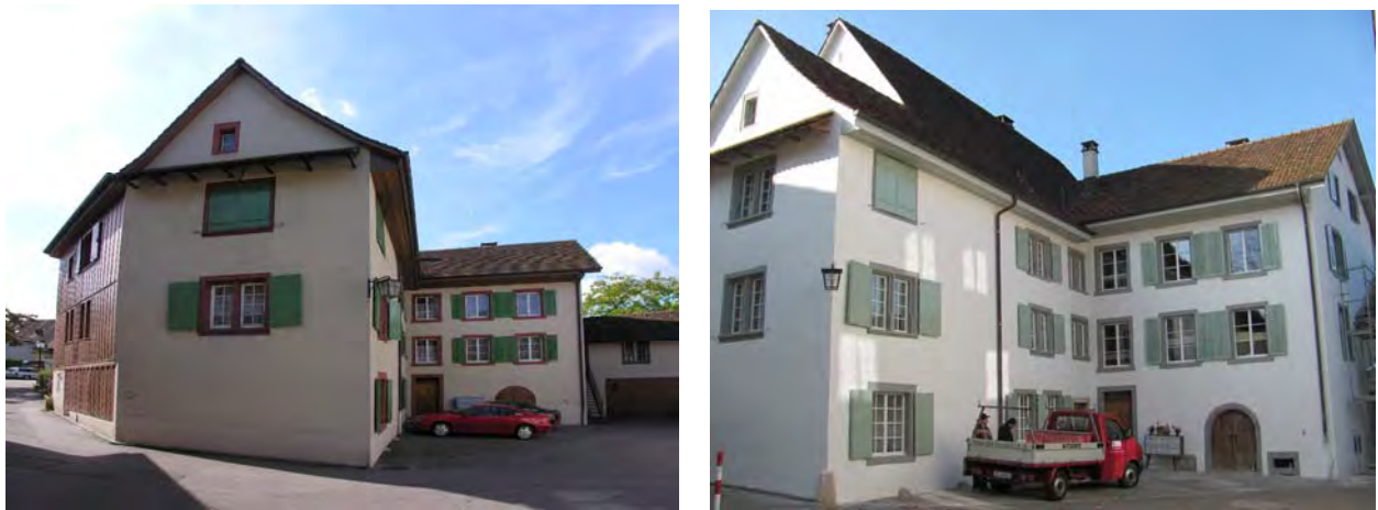
Figure 19: Historical building dating from the 14 th century that was renovated in Sissach (BL) with aerogel render in close corporation with the monument preservation authorities, before renovation and after renovation with approx. 6 cm aerogel rendering
