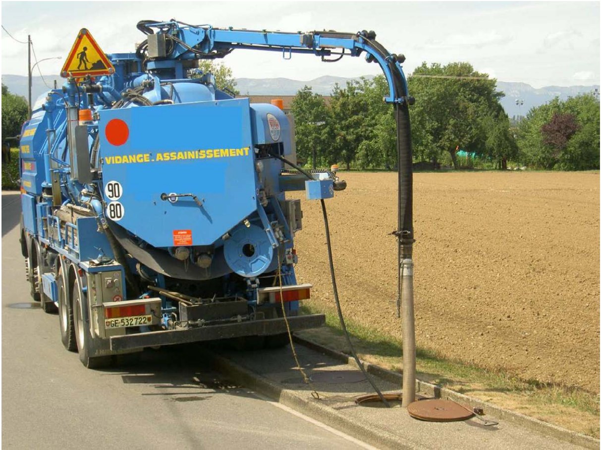
Fig. 3 – Sewer flushing
