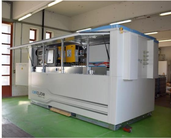
**Figure 2:** The all-vanadium RFB installed as the heart of the demonstration system in Martigny.
