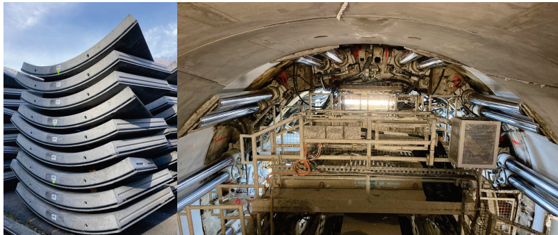
Fig. 1.1 - Stored segmental tunnel linings and installation of segments with TBM (author's own photographs).
