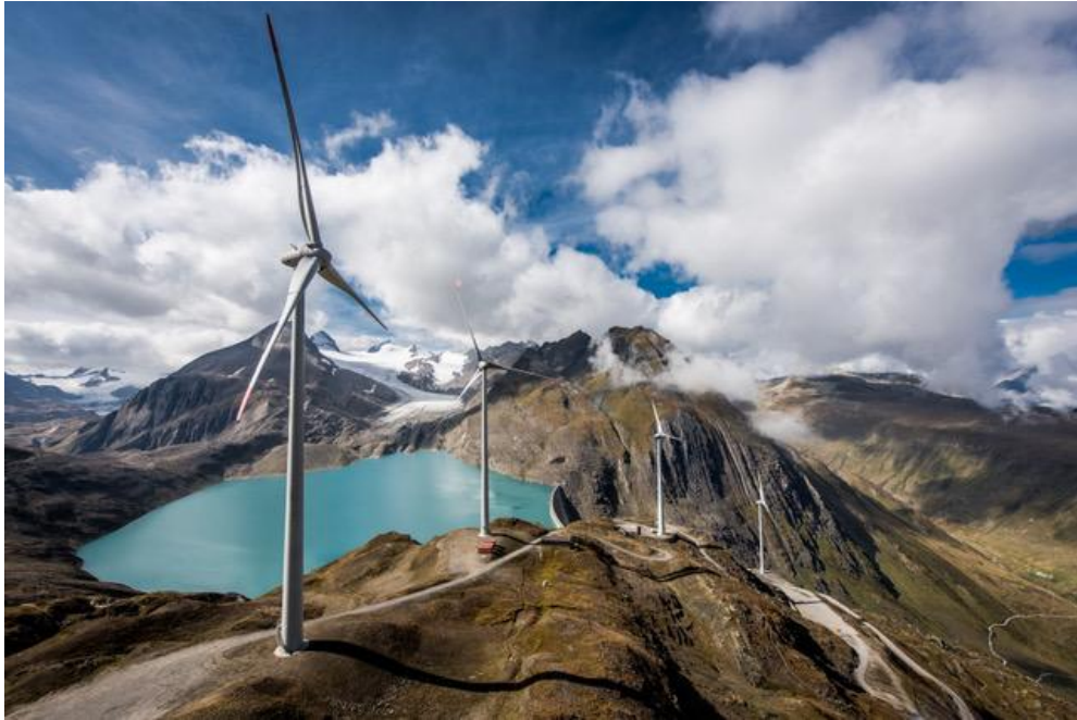
Figure 24: Wind turbine near the dam of Gries (source: Wikipedia).
