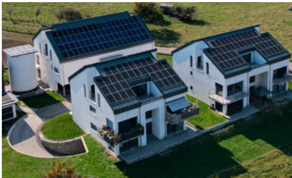
Figure 45: View of EcoThierrens, an eco-district located in Thierrens, in Switzerland.
