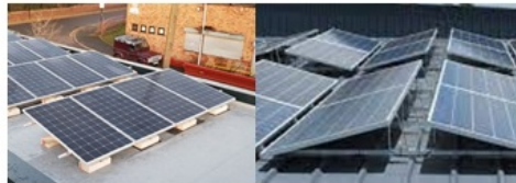
Figure A7: Panel arrangement according to portrait layout (left pane) and east-west structures (right pane).
