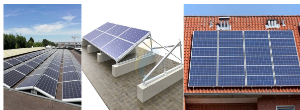
Figure 9: Panel arrangement for an east-west structure (left image), according to portrait layout (center image) and for the case of a slanted roof (right pane).
