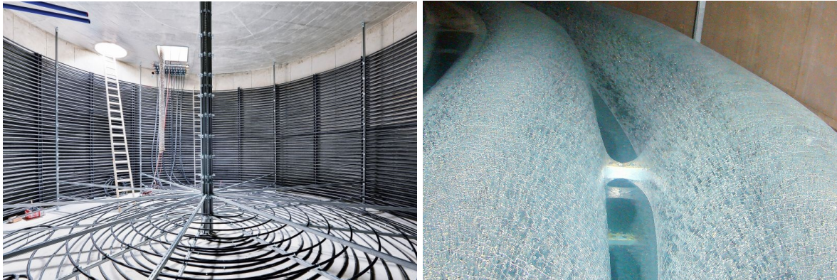
Figure 1: Ice-on-coil storage view from inside, in the left side picture. On the right side, the formation of an ice layer around the internal tubing inherently reduces thermal conductivity. Source: Viessmann.
