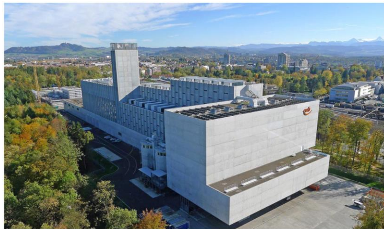
Figure 101 - Energy Hub at Forsthaus Bern
