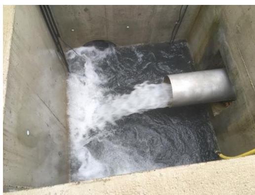
Figure 87 - Wellhead of GEO-01 producing thermal water containing a black-colored suspended load.
