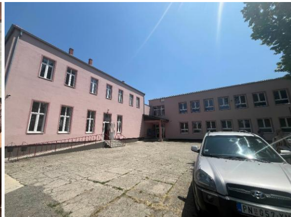
Refurbished primary school in Sikirica
