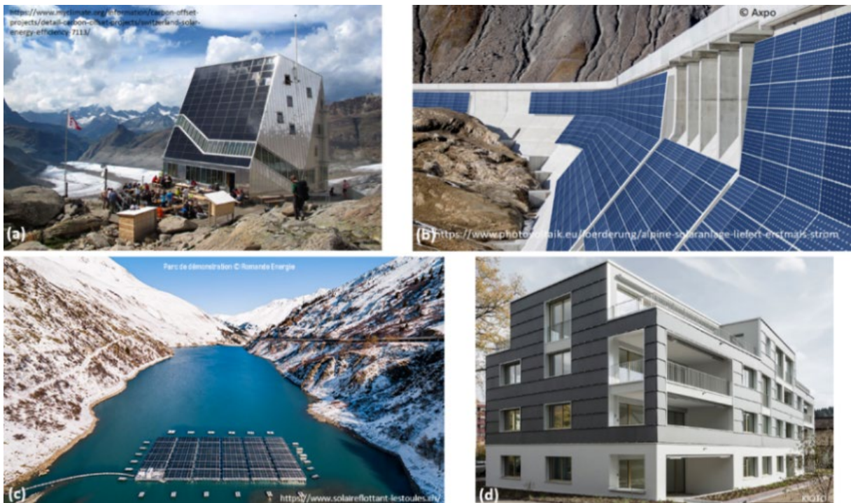
Figure 1: Examples of pilot projects for PV in an alpine environment: (a) "Monte Rosa SAC Hut", (b) 2.2 MW PV system dam Mutsee, (c) "Lac des Toules" in Switzerland and (d) BIPV (façade) system in Austria.
