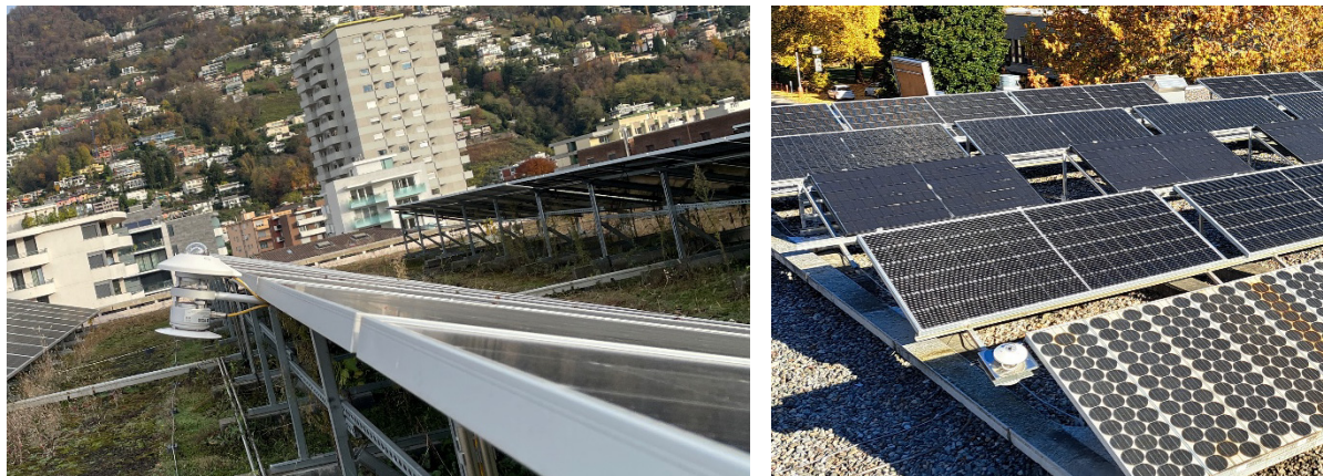
Figure 34: Placement of the G_{\text{POA}} and G_{\text{RPOA}} sensors at Viganello (left) and Trevano (right).
