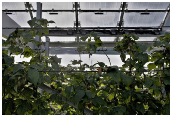
Figure 6: Illustration of the light transmission of the THEIA prototypes on crops in E-mode and MLT-mode, with photographs taken on the GEN1 installation.
