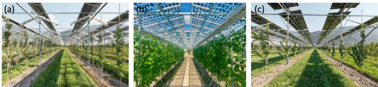
Figure 1: Possible implementation of agrivoltaic systems with spaced conventional modules, semi-transparent modules with partial cell coverage, and conventional modules on dynamic trackers. All photographs © Insolight 2025.
