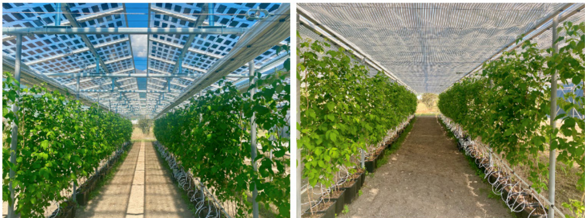
Figure 11: Second-generation (GEN2) agrivoltaic solution, with retracted (left) and deployed (right) shading screen.
