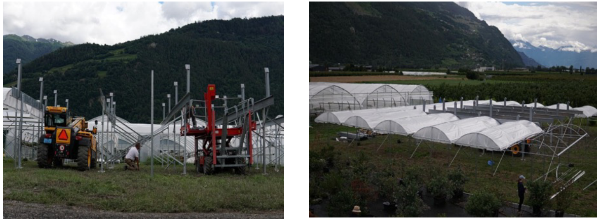
Figure 9: Photographs taken during the GEN1 prototype construction.
