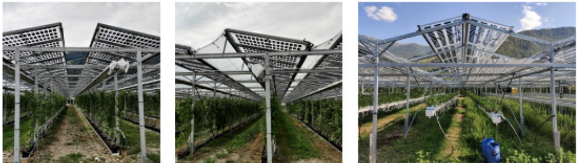
Figure 13: different modalities of the GEN2 commercial-scale agrivoltaic installation in Conthey. From left to right: (i) Raspberry part with East-West (EW) oriented modules. (ii) Raspberry part with West-only (WW) oriented modules. (iii) Strawberry part. Plastic tarps have been added during the year 2024 to close the gaps between modules and protect fruits against rain, except on the westernmost chapel of the strawberry zone to compare agronomic results with/without plastics between the panels.
