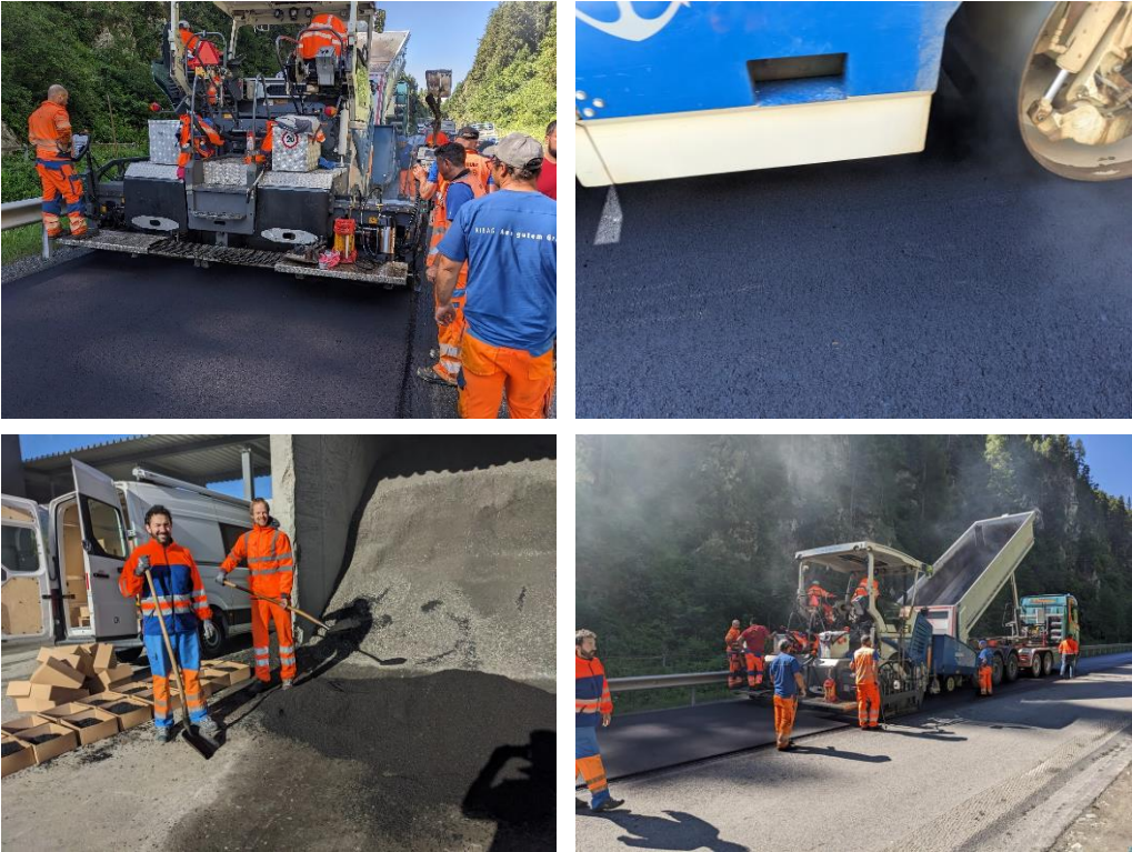
Figure 106: Construction of the AC 8 S pavement in the Charnadūra test section
