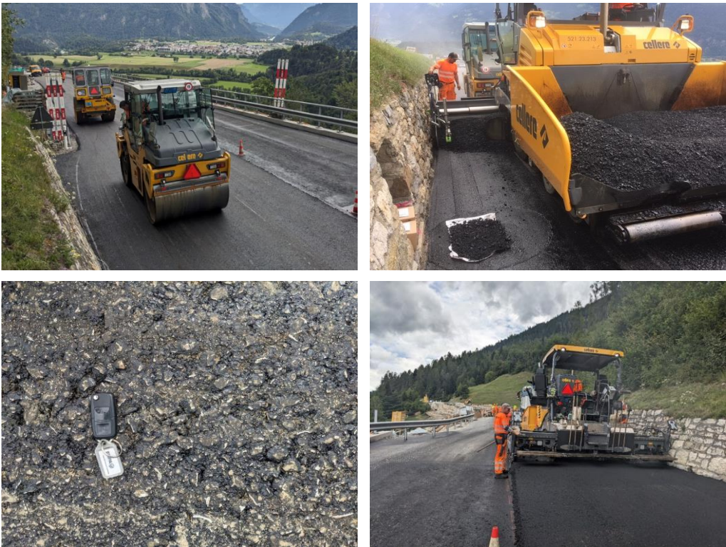
Figure 79: Construction of the AC T 22 S pavement in Tamins – Vel Mailens test section
