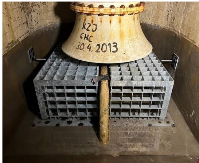
Figure 31: The grid installed on site underneath the booster pump bell.
