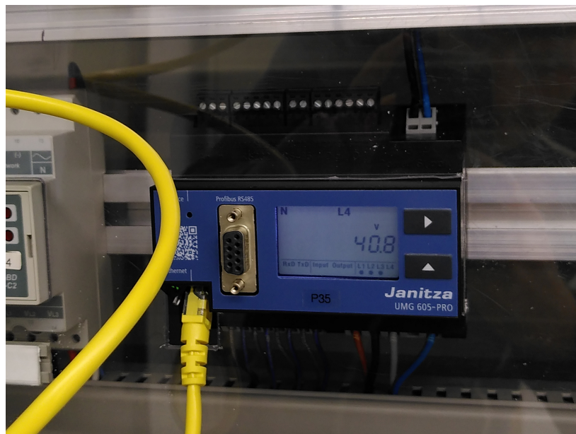
Figure 9. Janitza UMG-605 used for parking load monitoring.
