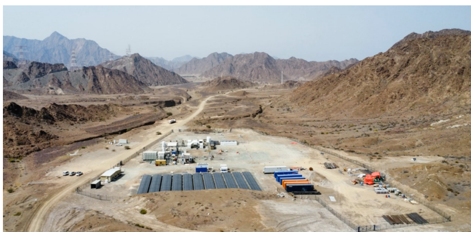
Figure 12. Site of the CO 2 injection project of the company 44.01 near Fujairah, eastern coast of UAE. The visible mountains are serpentinized peridotite. Solar panels (foreground) provide electricity for the operation. Image from 44.01 website.
