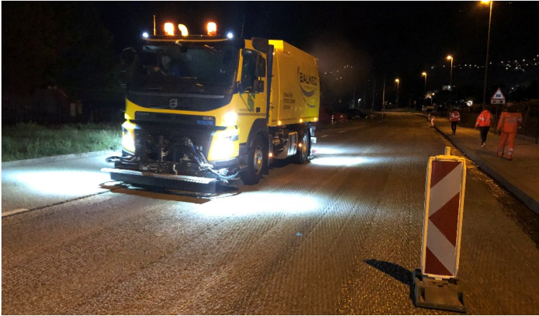
Figure 5: Dust cleaning of the milled surface
