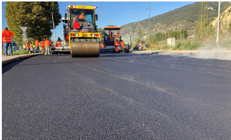
Figure 9: Placement of asphalt surface course
