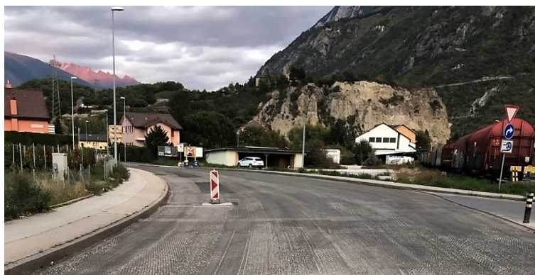
Figure 4: Milling of the existing surface of the test track
