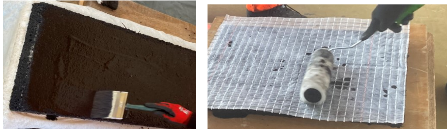
Figure 41: Application of System D
