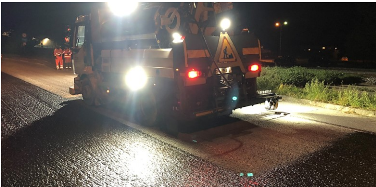
Figure 6: Spraying of the emulsion on the milled surface
