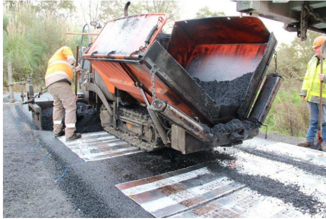
Figure 32: Installation of the test fields with asphalt reinforcement (Chazallon et al. 2019)
