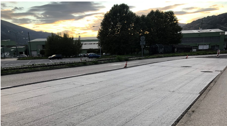
Figure 7: Laying of the grid reinforcement
