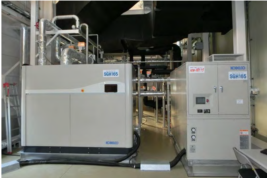
Figure 1: External appearance (steam compressor unit on the left, heat pump unit on the right)
