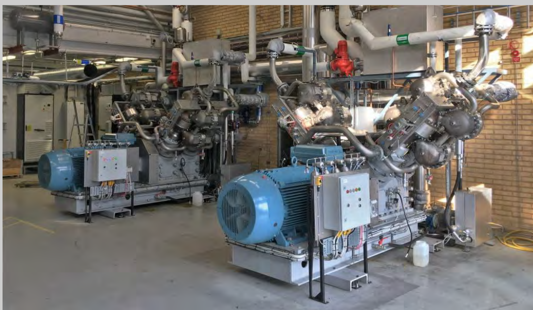
Figure 1: Two of the three heat pumps currently installed at AstraZeneca's R&D facility in Gothenburg, Sweden. Heat is transferred to the heat pump from the heat recovery circuit and steam is delivered from the heat pumps' steam generators to the steam distribution system. The third heat pump is installed on the opposite side of the room.
