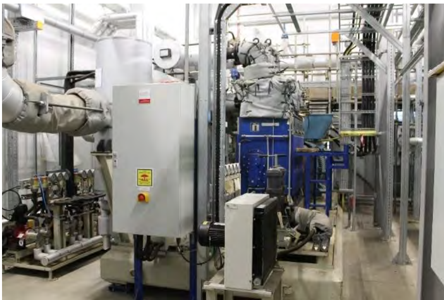
Figure 1: One of the two steam compressors installed at chemical plant, United Kingdom.
