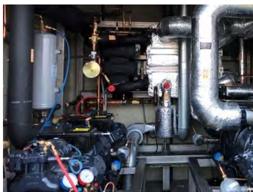
Figure 1: SkaleUP cascade HTHP installed in 10 feet container, Trondheim Norway
