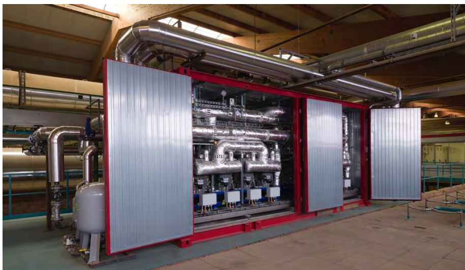
Figure 1: DryFiciency Heat Pump at Wienerberger brick production facility in Uttendorf, Austria
