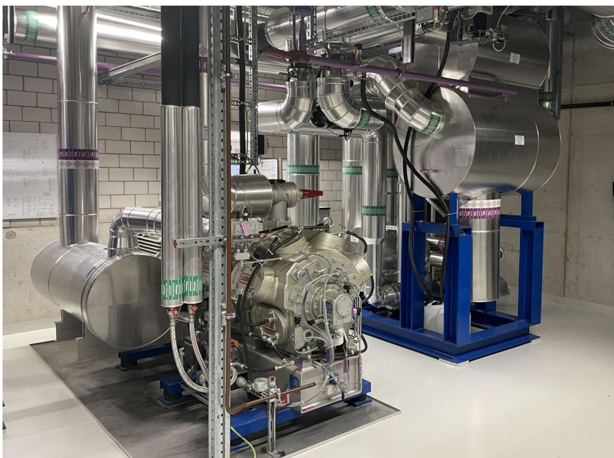
Industrial heat pump integrated in the energy centre of a Swiss company (Photo: C. Arpagaus, OST, 4 June 2024)
