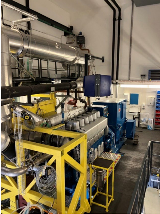
Figure 12: Pilot Plant Building (June 24)
