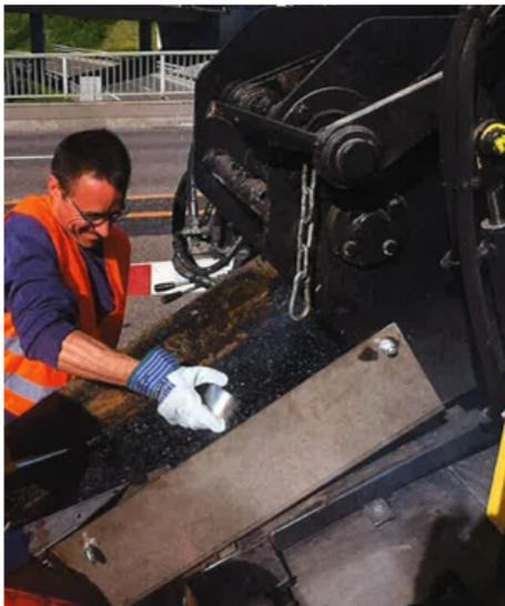
Figure 8 - Production of the test specimen on the construction site
