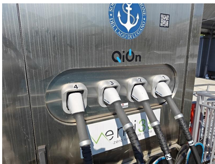
Figure 20 - The 4 400A charging cables of the fast-charging station
