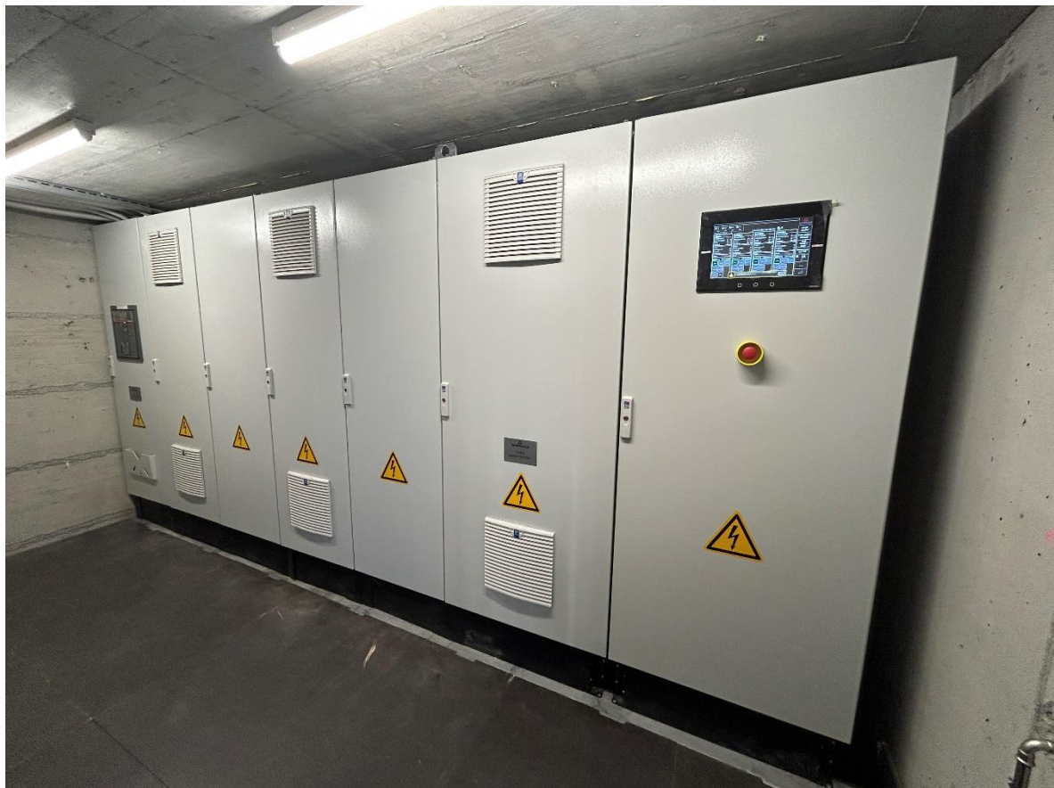
Figure 19 - The electrical system inside the structure at the pier with the charging control interface
