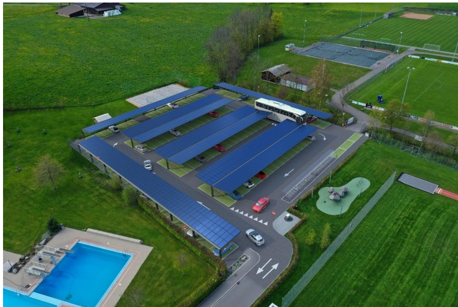
Figure 3. Visualization of one project scenario of a photovoltaic system above a car parking in Wittenbach (Pröschel et al., 2023). The rated power of the variant of PV system depicted here amounts to 449 kWp.
