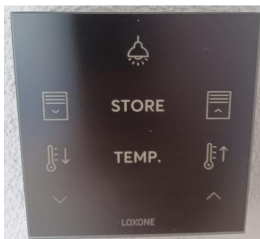
Figure 7: Loxone Touch pure flex in the pilot site
