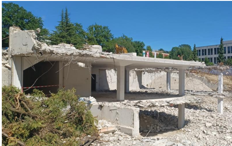
Figure 28 : View of the MixCity building during the combined deconstruction and demolition © Julien Pathé 2401
