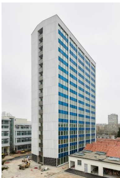
Figure 25 : View of the tower 107 in the PPN project
