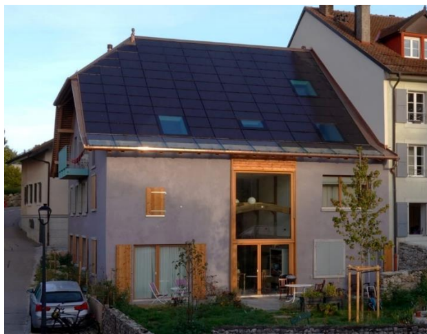
Figure 22 : View of the Chauchy building
