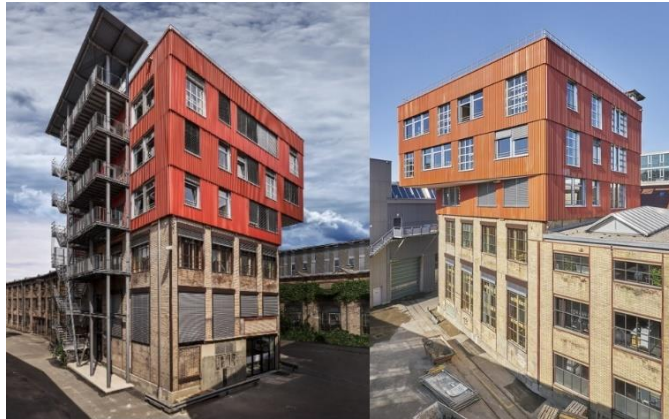
Figure 9 : View of the K.118 building
