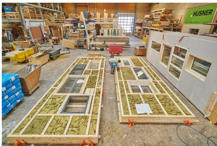
Figure 20 : View of the prefabricated façade of Elys during assembling the workshop (top) and during the construction on site (bottom)
