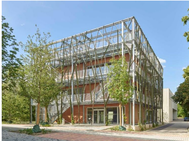
Figure 15 : View of the Primeo Energie Kosmos building © Beat Ernst
