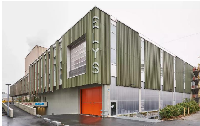
Figure 18 : View of the Elys building
