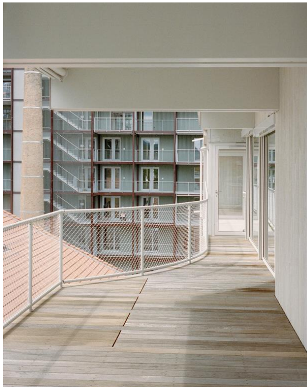
Figure 13 : View of a balcony of the Hobelwerk Haus D building showing the reused wooden floorboards.
