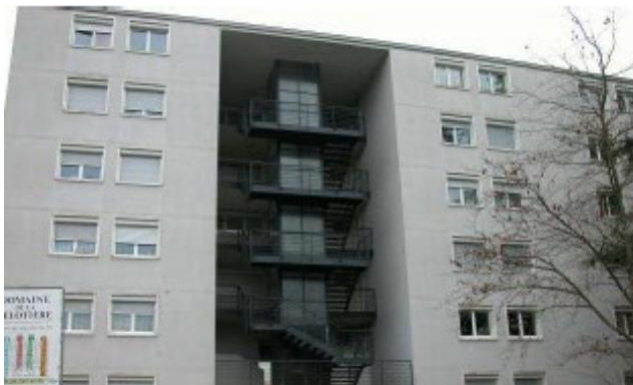
Figure 27 : View of the Fayard building
