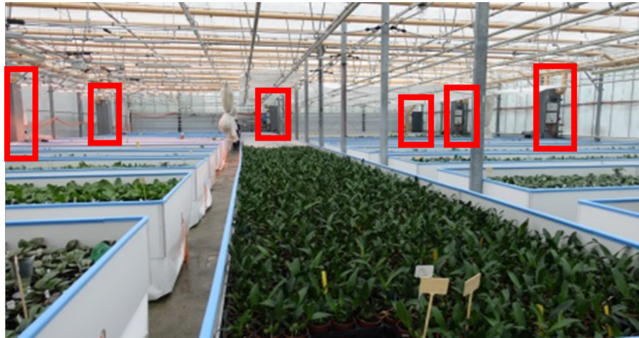
Figure 19: Demonstrator greenhouse with the desorbers in red.
