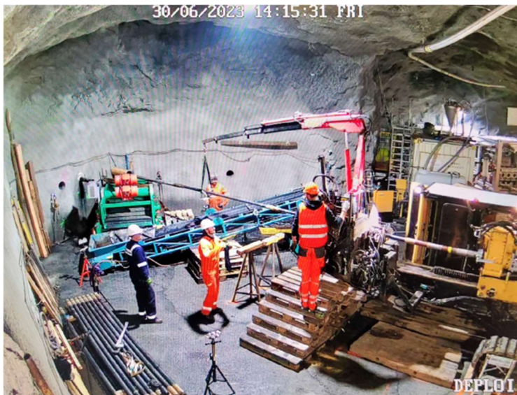
Figure 18. Rig repositioned for drilling through stove pipe 2.
