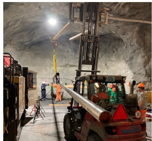
Figure 7: Overview of the drill site (left) and making-up and running-in-hole the 'empty' DSSD drilling assembly without electronics (right) for test purposes.
