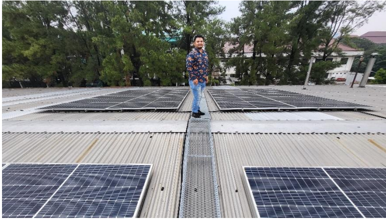
Polytechnic Jakarta, solar PV installation of lab rooftop
