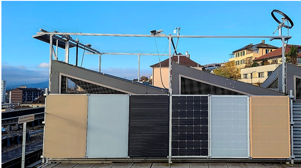
Fig. 31 Demonstrator site on microcity rooftop at Neuchâtel, Switzerland
