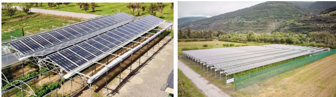
Figure 14: Photographs of the projects based on the new generation Insolagrín solution in Conthey. Left: 16kWp demonstrator. Right: 265kWp commercial-scale installation with dedicated parts optimized for the cultivation of raspberries and strawberries.
