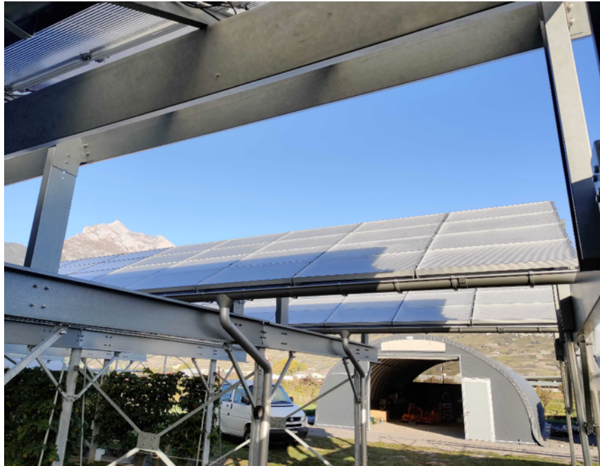
Figure 27: Example of frost on the panels in early morning. Frost and condensation act as absorbers and diffusers, thus lowering the amount of light reaching the solar cells.
