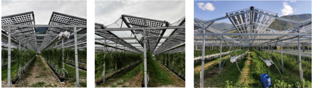
Figure 15: different modalities of the new generation commercial-scale agrivoltaic installation in Conthey. From left to right: (i) Raspberry part with East-West (EW) oriented modules. (ii) Raspberry part with West-only (WW) oriented modules. (iii) Strawberry part. Plastic tarps have been added during the year 2024 to close the gaps between modules and protect fruits against rain, except on the westernmost chapel to compare agronomic results with/without plastics between the panels.
