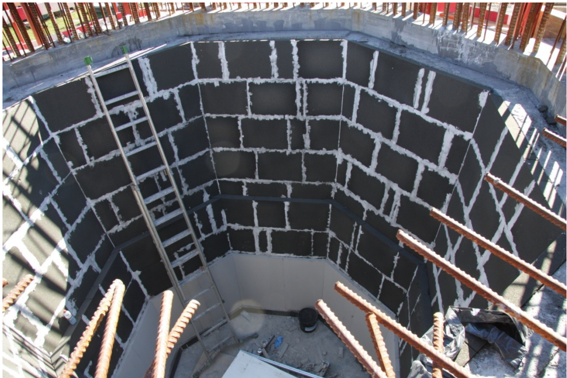
FIGURE 6: INTERNAL PART OF THE NEW STORAGE PROTOTYPE.
