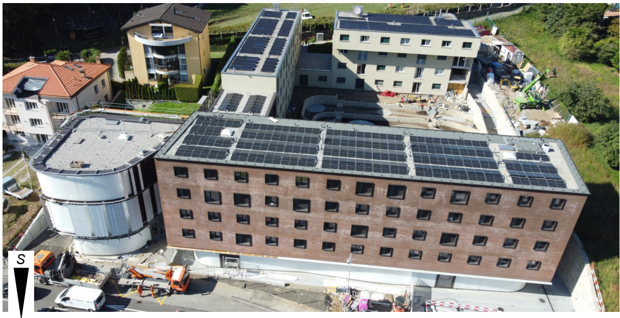
Figure 1: Franklin University Campus in Sorengo; the BIPV system is installed on the new auditorium's facade on the complex's west side.
