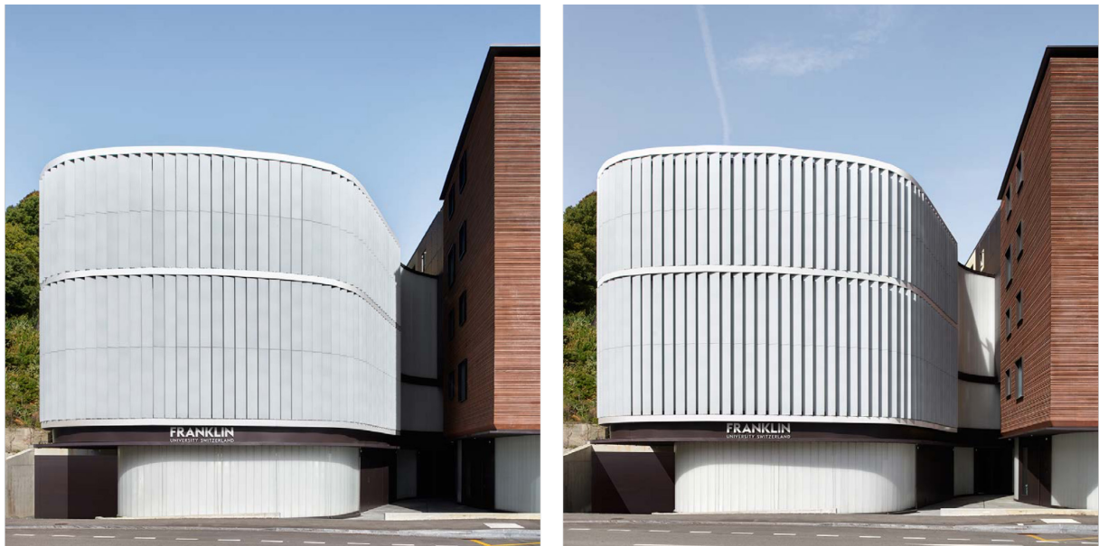
Figure 2: Franklin University Auditorium. Two different configurations of the shading system. Source: Flaviano Capriotti Architetti.
