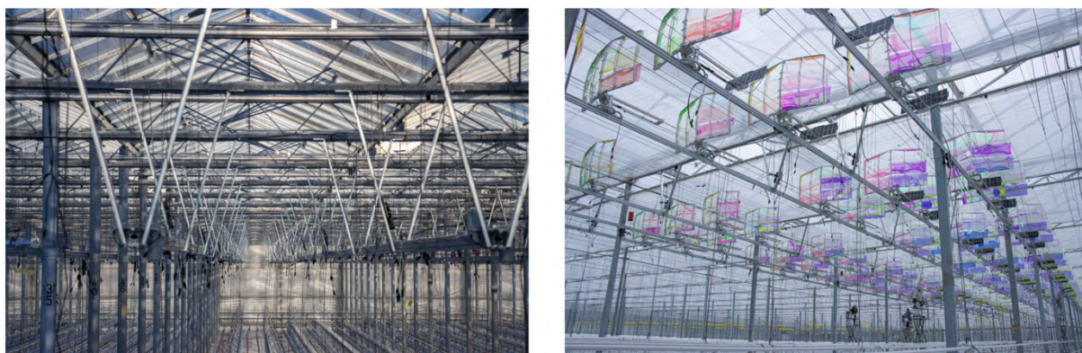
Figure 9 - Images of the holding structure at Serre des Marais.
