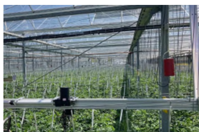
Figure 22 - Motors installed on the profiles.
