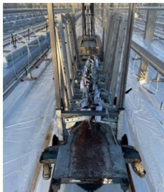
Figure 23 - Mechanisms on the trolleys, ready to be installed on the profiles.
