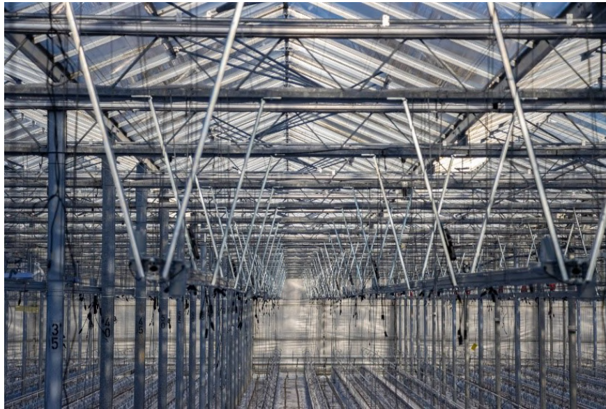
Figure 21 - V-structure and profiles installed along two cultivation lines.
