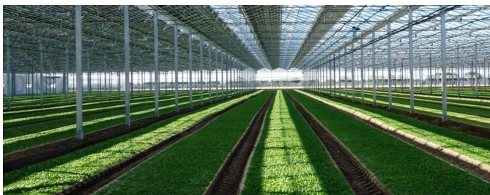
Figure 1 - Greenhouse using standard solar modules covering 50% of the roofing (South side). High light losses and light level inhomogeneities results from the APV deployment.
