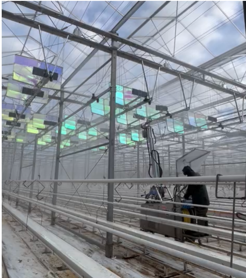
Figure 13 - Cleaning of the installation using the Aquajet machine (high-pressure cleaning).
