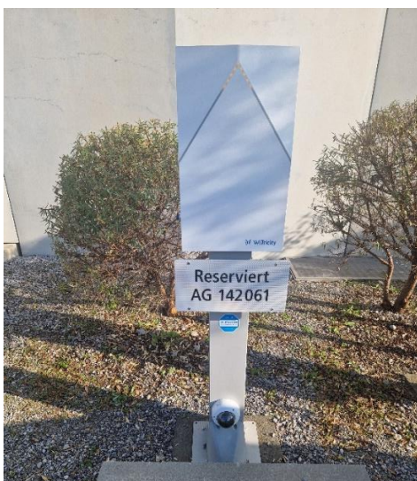
Abbildung 5: WiTricity Halo Wireless Charger 11 kW Wall Box
