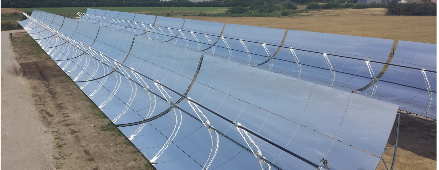
Two collector rows of the parabolic trough collector field in Brønderslev, DK. The 16.6MW th -Plant has an aperture area of 29'929 m 2 and is combined with a biomass-organic rankine cycle for combined heat and power generation. Foto: Brønderslev Forsyning.
