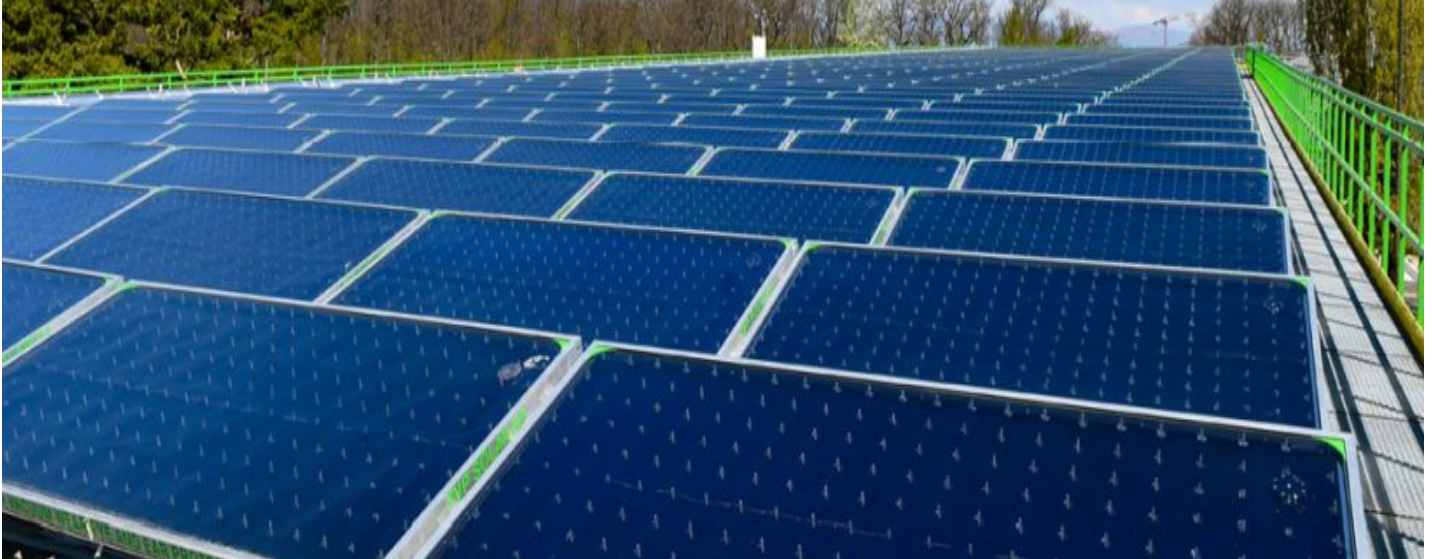
Vacuum flat plate collectors provide heat for the district heating network of Geneva. Source: TVP Solar
