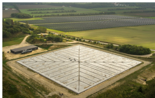
Pit thermal energy store of Dronninglund (DK), the large solar thermal field installation can be seen in the background.
