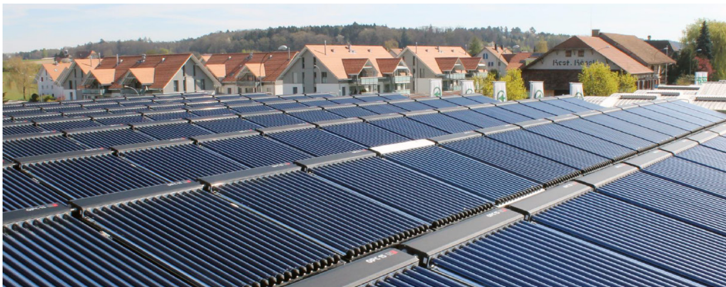
Evacuated tube collectors provide heat for the network of WLS in Schüpfen CH.
