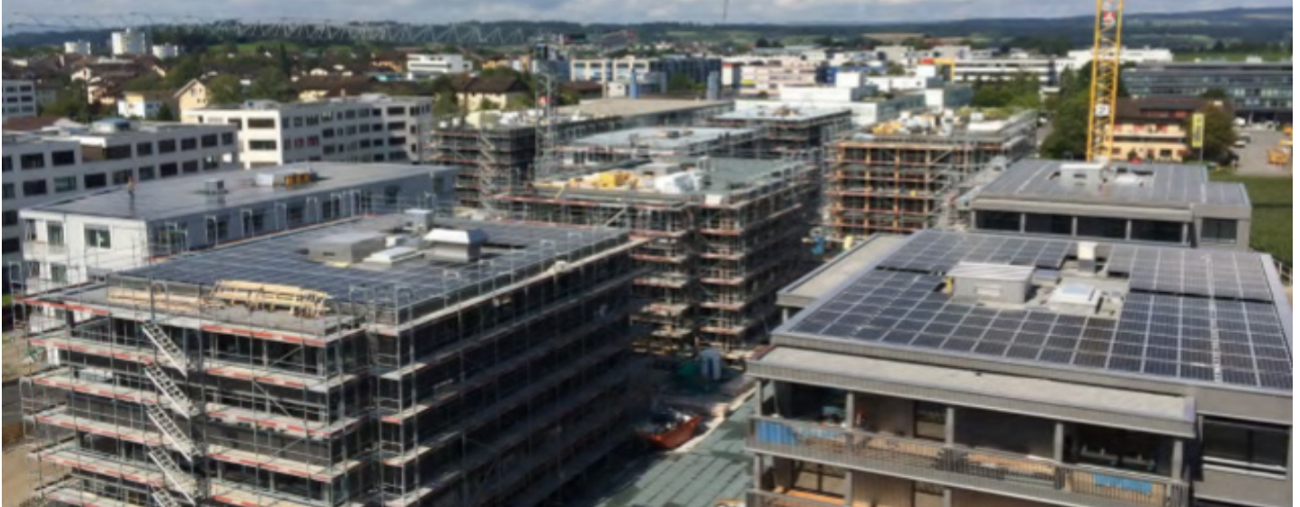
Switzerland's largest solar thermal installation consist of about 3500 m 2 of PVT collectors regenerating borehole storages of the lowtemperature network for the Suurstoffi blocks.
