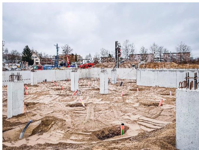
Figure 8: HT-BTES during the construction phase. The heads of the boreholes are clearly visible. Also visible, one third of the BTES is situated below the new parking slot. Picture from Kevin Olas.
