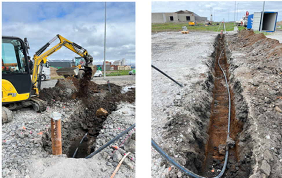
Figure 15: The trenches for burying water tubes and electrical cables extend from the miniRUEDI site to Carb2 (left) and Carb3 (right) wells.
