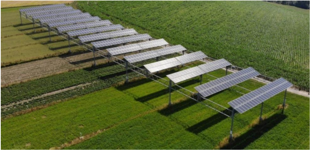
Figure 2: System example for "open arable crop" management status. Agri-PV trial system (APV Resola) with non-tracking modules in Heggelbach (Germany). The modules are installed at a height of 5.5 m and the distance between the supports in the longitudinal direction is 19 m (Hofgemeinschaft Heggelbach, n.d.).
