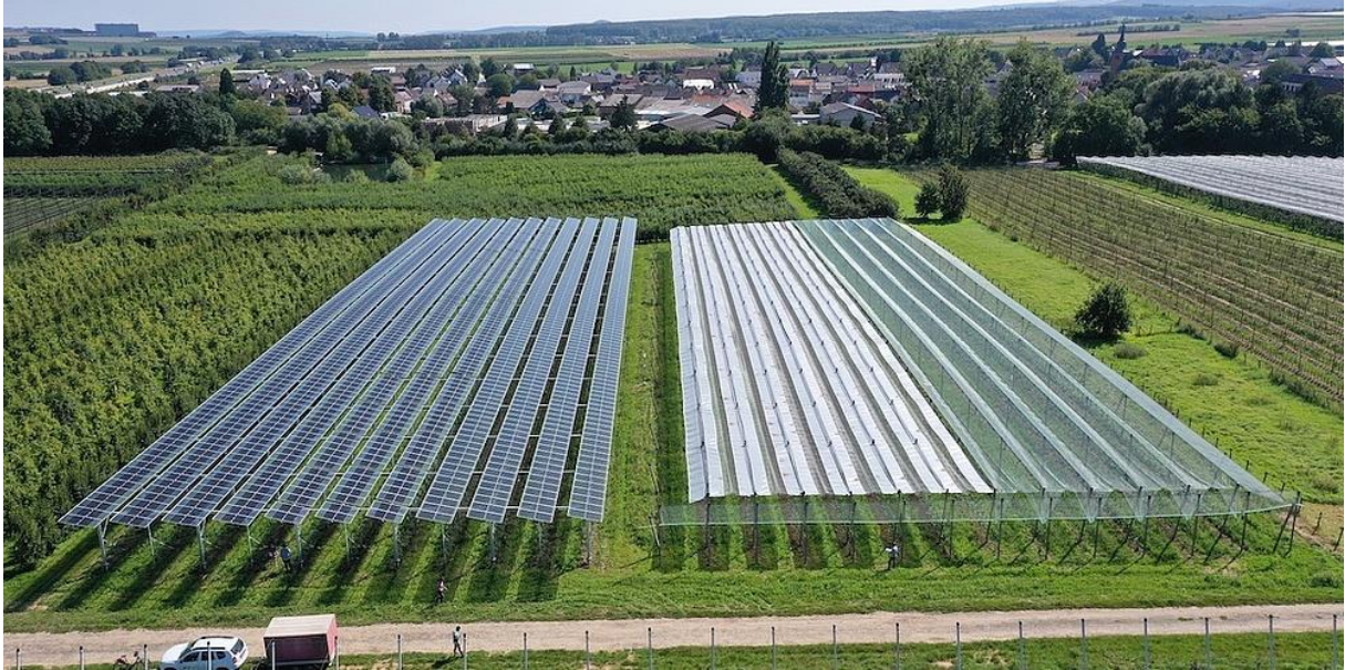
Figure 4: System example for "permanent crops" and "protected cultivation" management status. Agri-PV system above an orchard in Gelsdorf (DE). With the APV system (left in the picture), the existing crop protection measures (right in the picture) could be substituted (Energy experts, n.d.).
