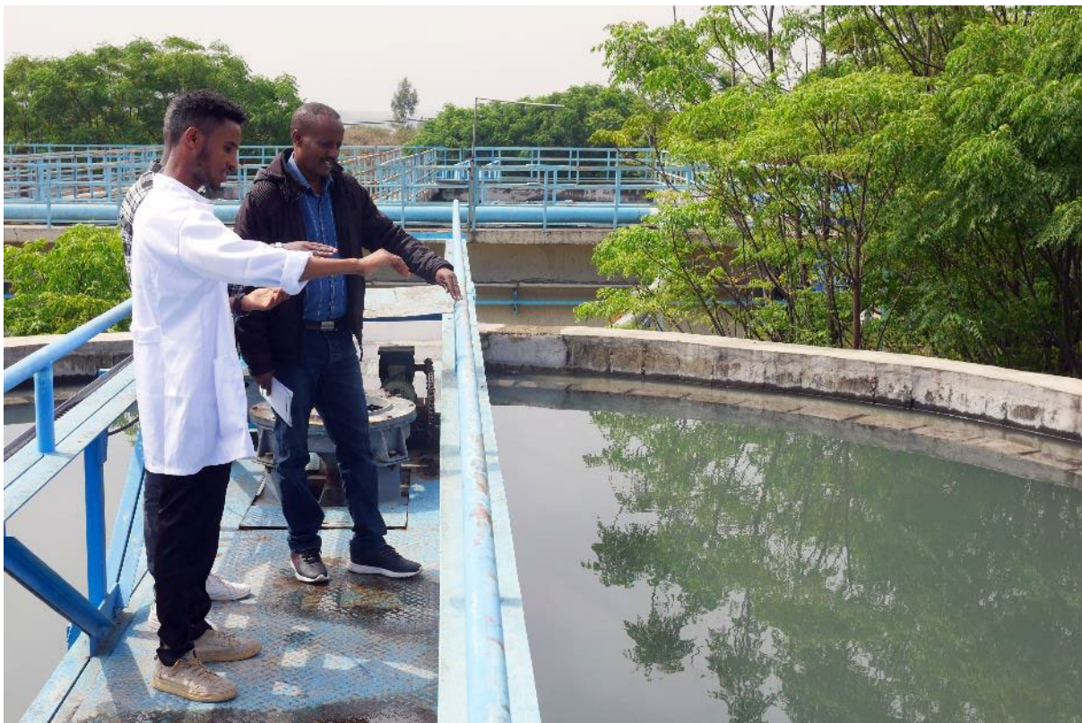
Wastewater treatment operated by the industrial park, treating effluent from 3 garment factories
