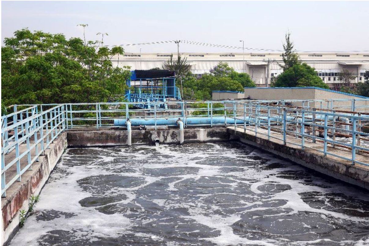
Wastewater treatment plant, factory shed in the background
