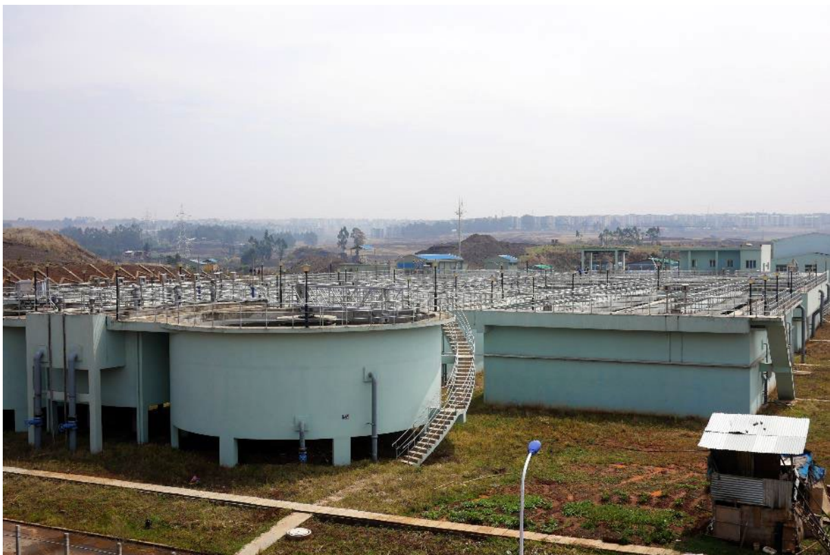
New wastewater treatment plant (not yet operational) for the expansion of Bole Lemi Industrial Park
