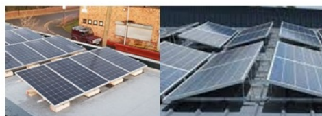
Figure 15: Panel arrangement according to portrait layout (left pane) and east-west structures (right pane).
