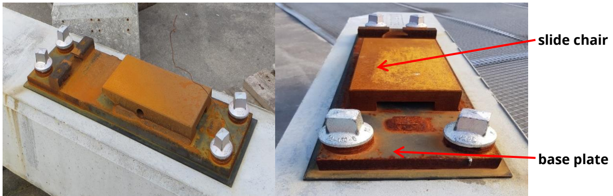
Figure 21:base plate and slide chair mounted on a concrete sleeper
