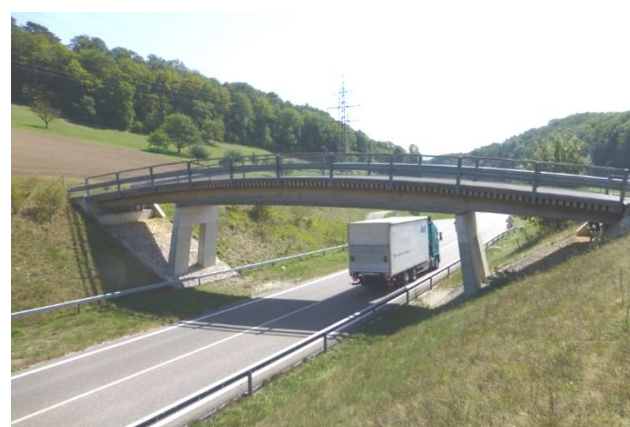
Figure 9: The monitored Horen bridge close to Aarau that crosses a road, photographed from the north side. The width of the load-bearing beams is about 1600 mm.
