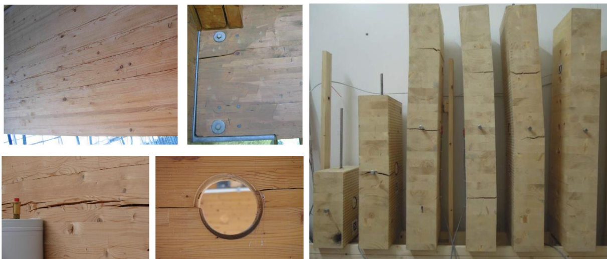
Figure 3: Cracked unreinforced glulam beams (top) free shrinkage with smaller cracks (top left), deep shrinkage cracks between fasteners (top right) and cracks in reinforced glulam beams (bottom), Dietsch (2017)
