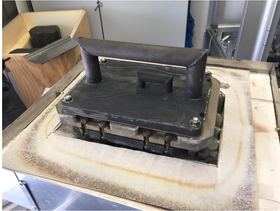
Figure 27: The bypass installed inside the StackBox in 2021
