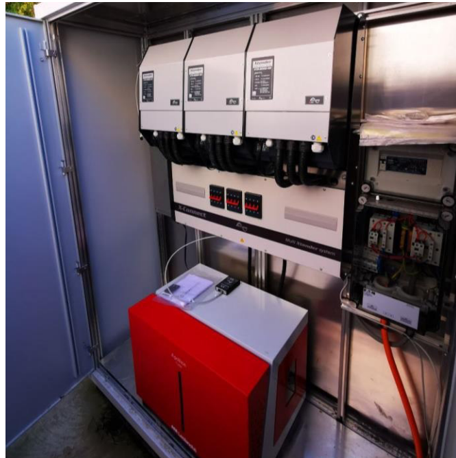
Figure 10: Site 4 - OIKEN Box containing the solarlog and the control box that allows data recovery
