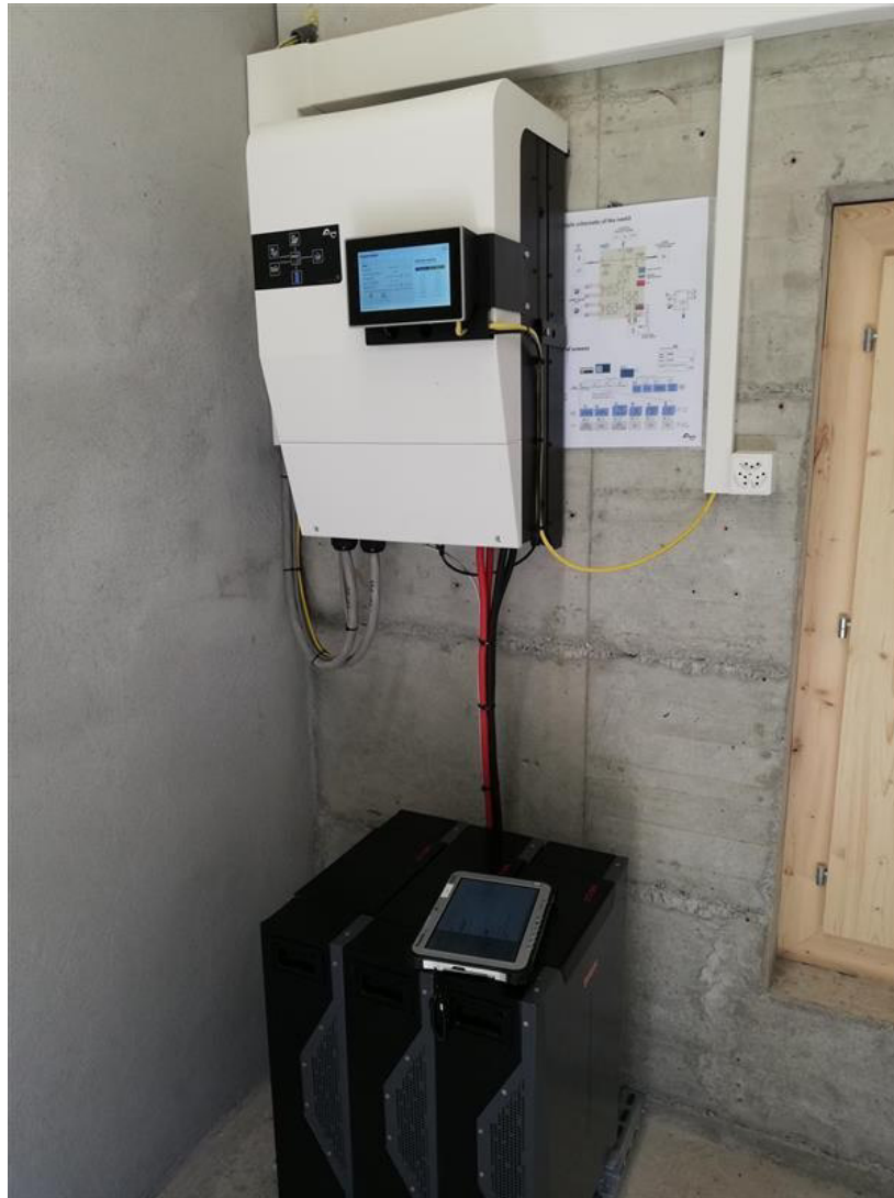
Figure 6: Next3 inverter at the FMA site in Gryon
