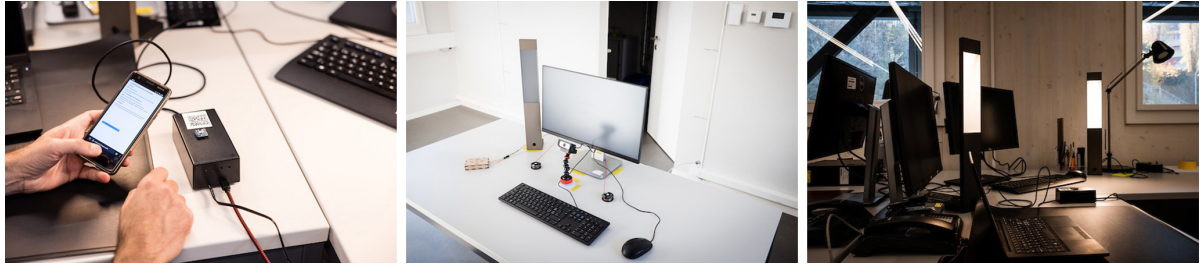
Figure 3. Task lighting fixture and operation. From left to right: the presence activation procedure, the task lighting setting on the occupant's desk, and a view of its use on evenfall exterior lighting conditions.
