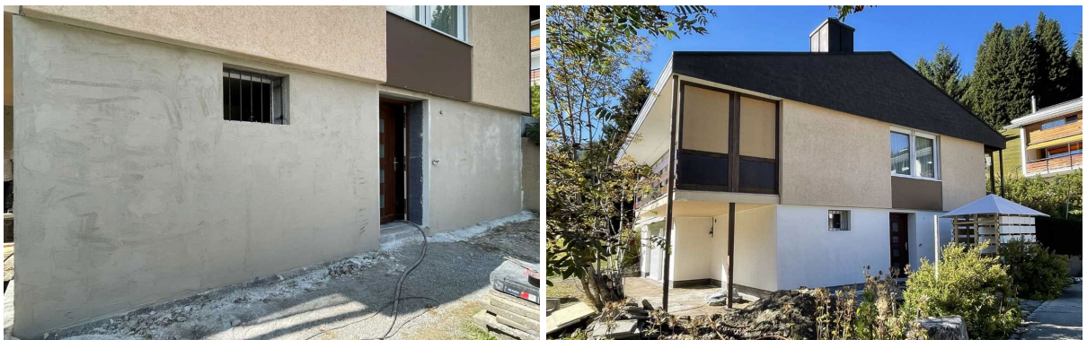
Figure 63. Left: View of the façade with the adhesive mortar applied. Right: View of the villa with the rough coating applied.
