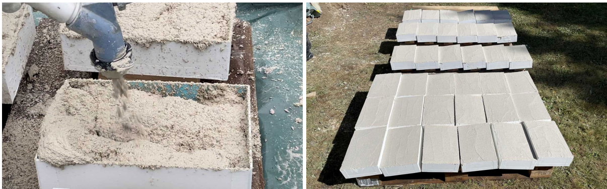
Figure 33. Left: Insulating render 1 begin applied. Right: Plates with adhesive mortar applied.
