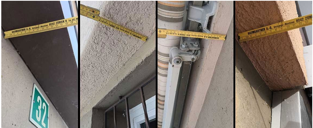
Figure 7. On-site check of the façade and the available space for installing the thermal insulation.
