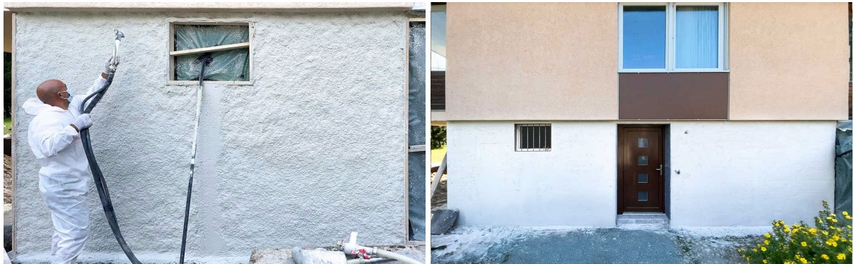
Figure 59. Left: Application of the insulating render (2) on the façade. Right: View of the façade with the insulating render applied and the surface smoothen.
