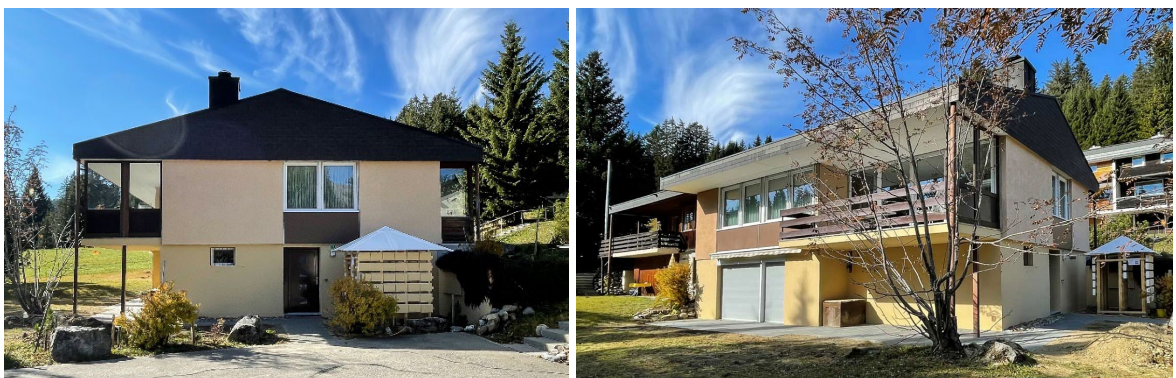
Figure 64. View of the final state of the renovated villa.
