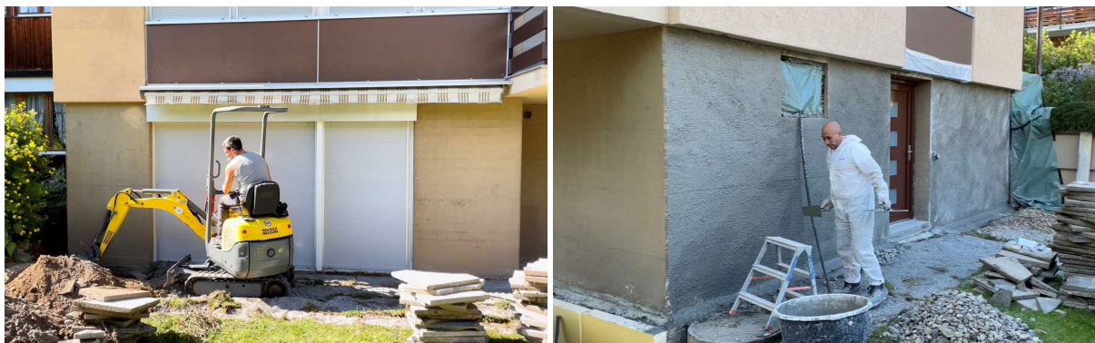
Figure 58. Left: Excavation of the trench around the villa for the application of XPS for breaking the thermal bridge. Right: Application of the pre-spray mortar on the façade.
