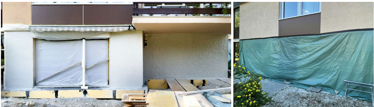
Figure 60. Left: View of the façade with the insulating render applied and the surface smoothen. Right: Plastic foil applied on the façade to prevent early drying during the hardening process.
