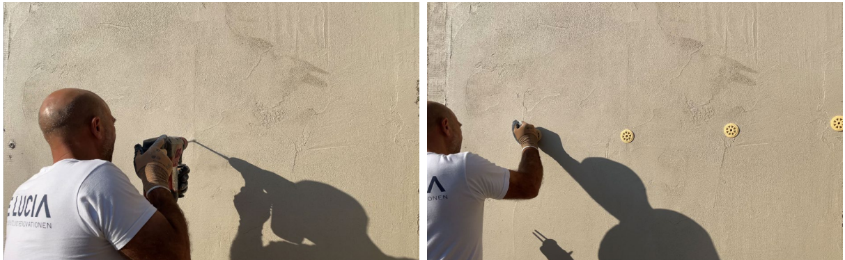
Figure 62. Left: Application of the anchor system.
