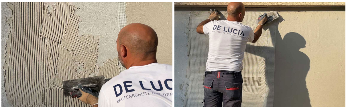
Figure 61. Left: Application of the adhesive mortar on top of the insulating render. Right: Application of the net embedded into the adhesive mortar.
