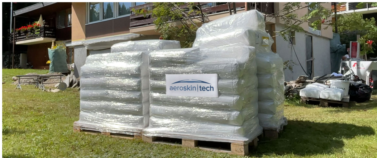
Figure 13. Some of the bags of the insulation renders to be applied in the façade and the testing plates.
